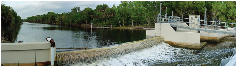
Top: A conceptual diagram illustrating water cycle processes included in the local scale model. Bottom: An intricate system of canals, weirs, and ponds are operated seasonally to shunt water off the land to prevent flooding in the summer, and hold back water to recharge aquifers in winter.
