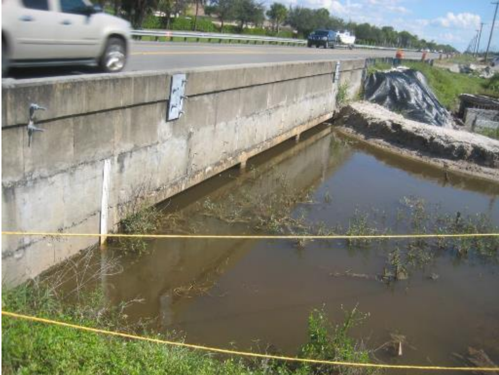
Figure 4.9. Existing Cross-Drain under U.S. Highway 41 at Throat Canal
