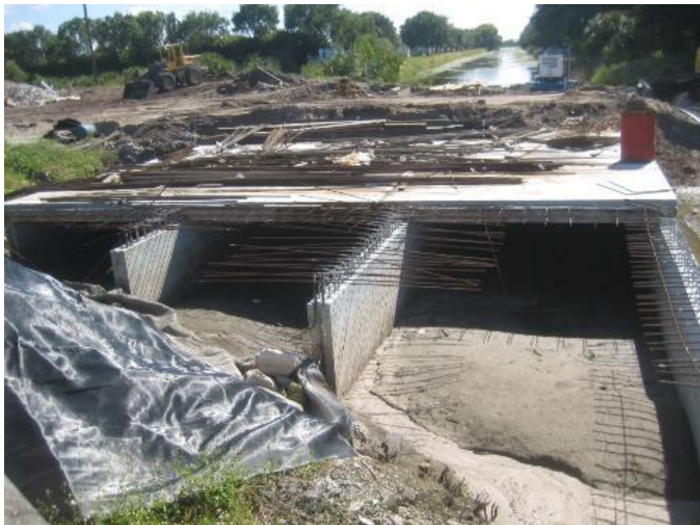
Figure 4.10. Current Construction of Cross-Drain under U.S. Highway 41 at Throat Canal.
