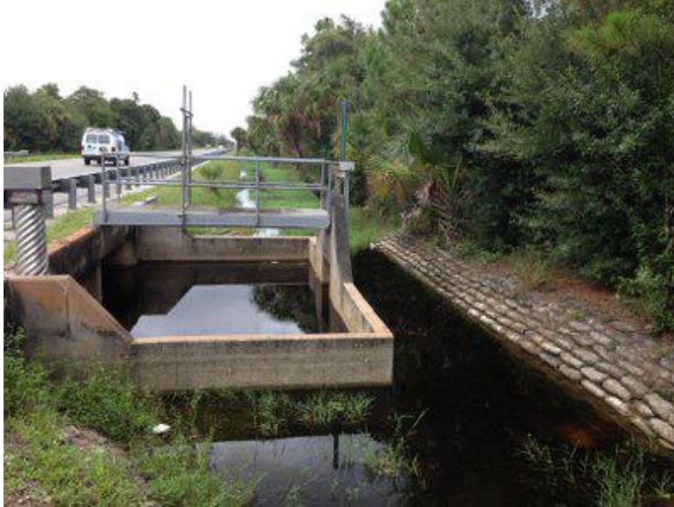
Figure 16. TAMIEHEND Structure Looking North (06/26/2013) Note: Belle Meade Flow-way To East
