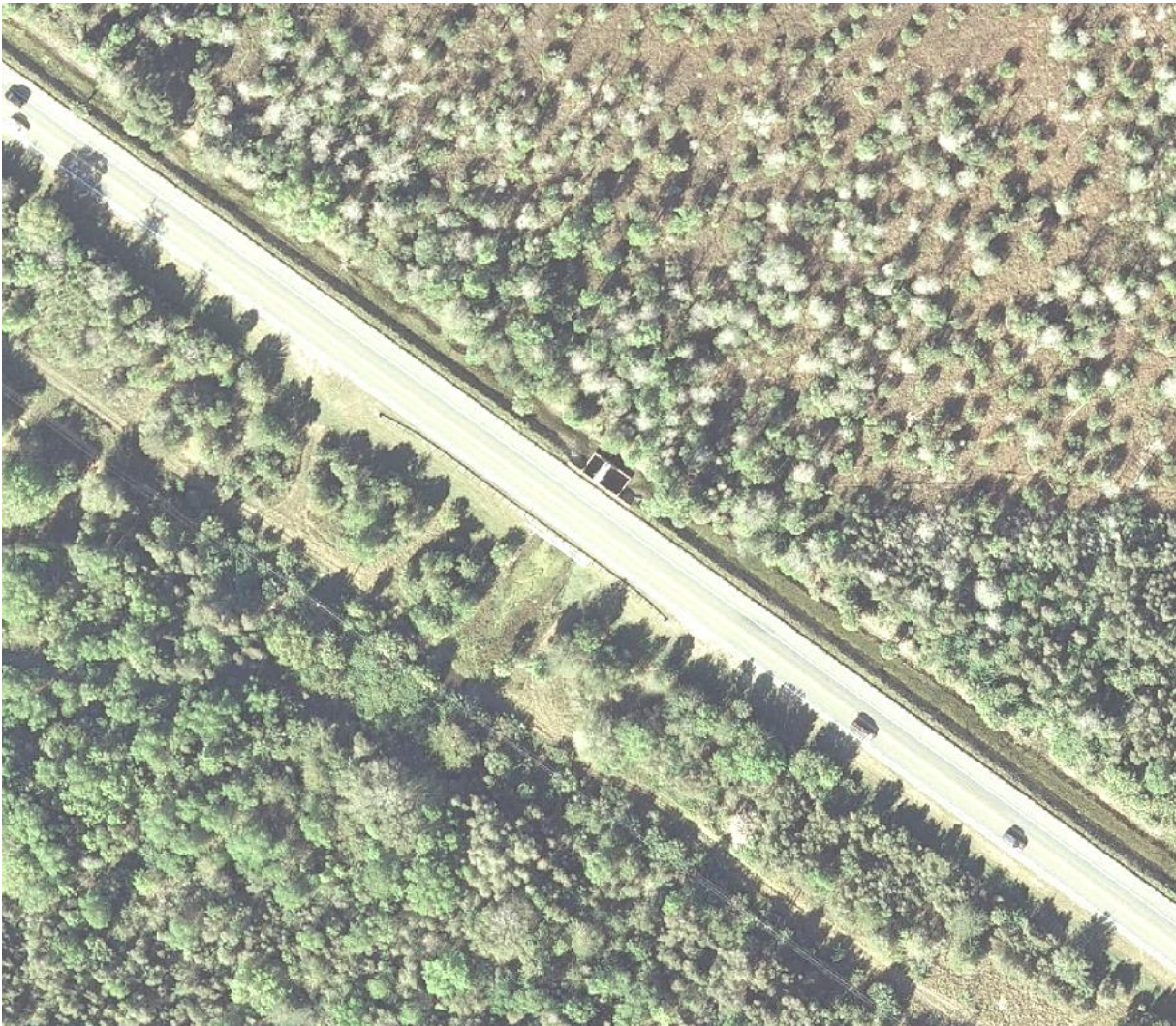
Figure 18. TAMIHEND Structure At US41/Tamiami Canal Henderson Creek East Branch Headwaters
