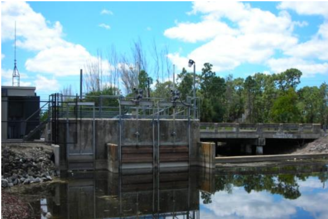
Figure 14. Upstream view of Henderson Creek Control Structure No.1 Showing Ogee Weir, Automated Sluice Gates, and Manual Sluice Gate (Photo Courtesy: SFWMD)
